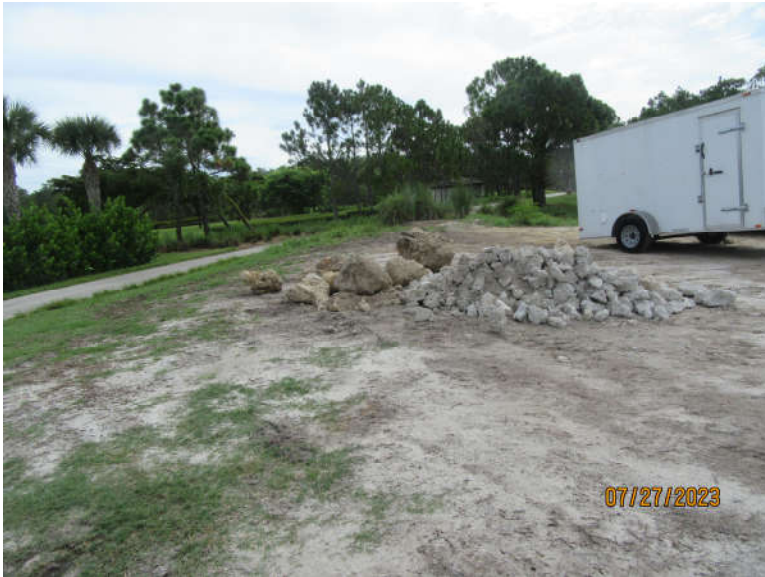
Large boulders moved to storage area
