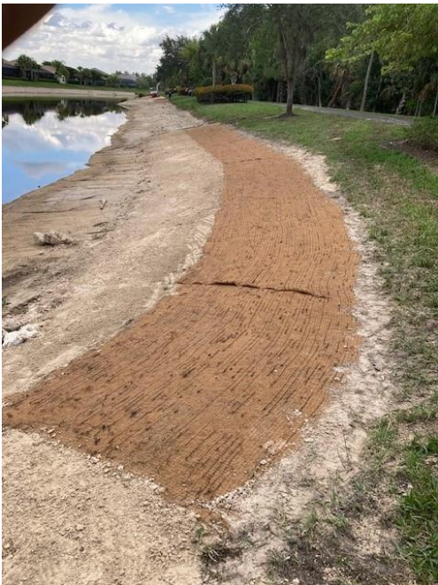
Monday, June 19, 2023, Quarry Dr, runoff from walking trail repaired, Lk 36a.
