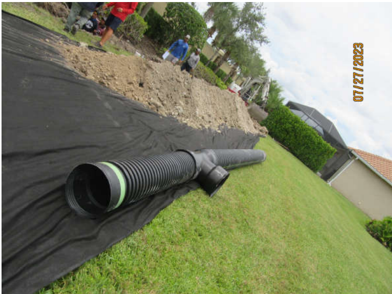
Thursday July 27 th – Excavation activities
